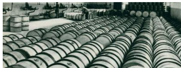
Keg filling line: Lubricating oil for Army, Air Force and Navy.
